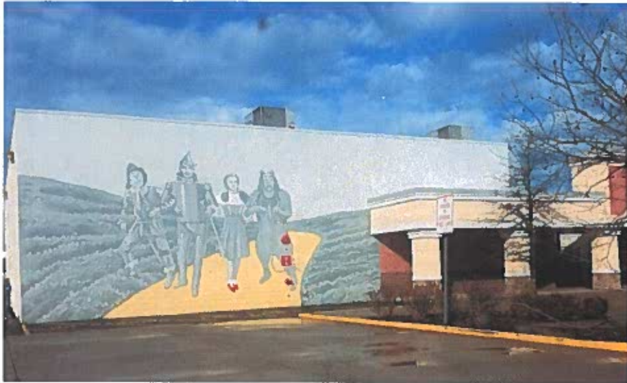
Illustration 5 – Premiere Cinemas Creative treatment of large expanse of blank wall
