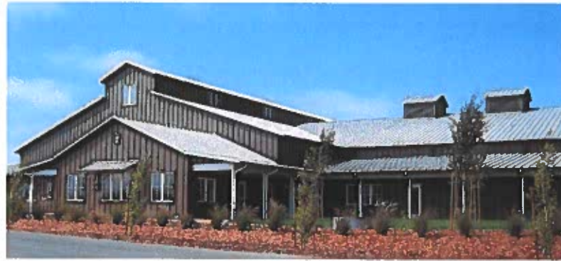
Illustrations 19 and 20 – PNC Bank, Virginia and Winery, Massachusetts Examples of new construction with clerestory elements
