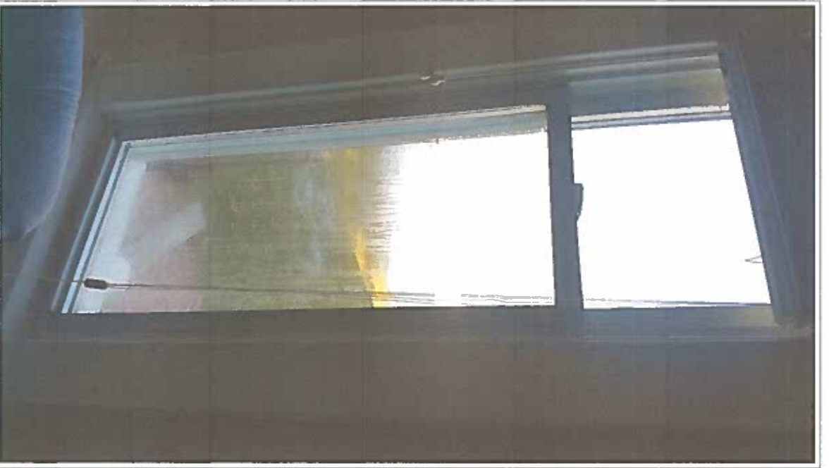
This is the inside view of an existing window.
