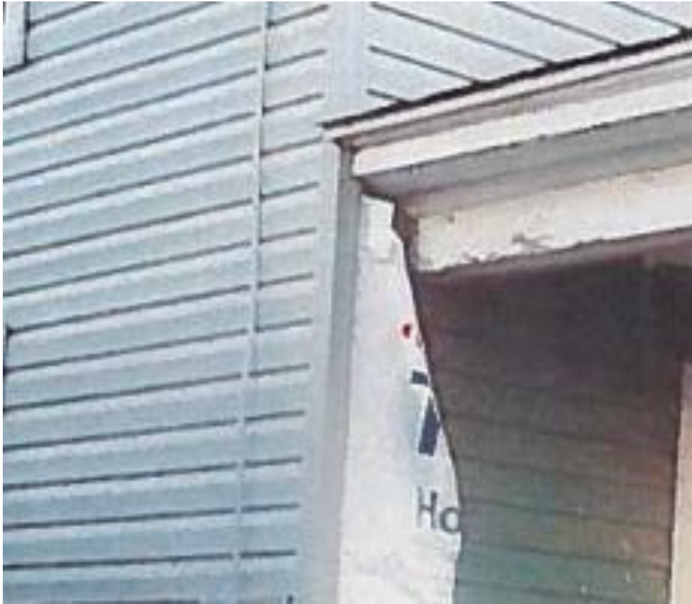
New Siding with Original Siding Exposed
