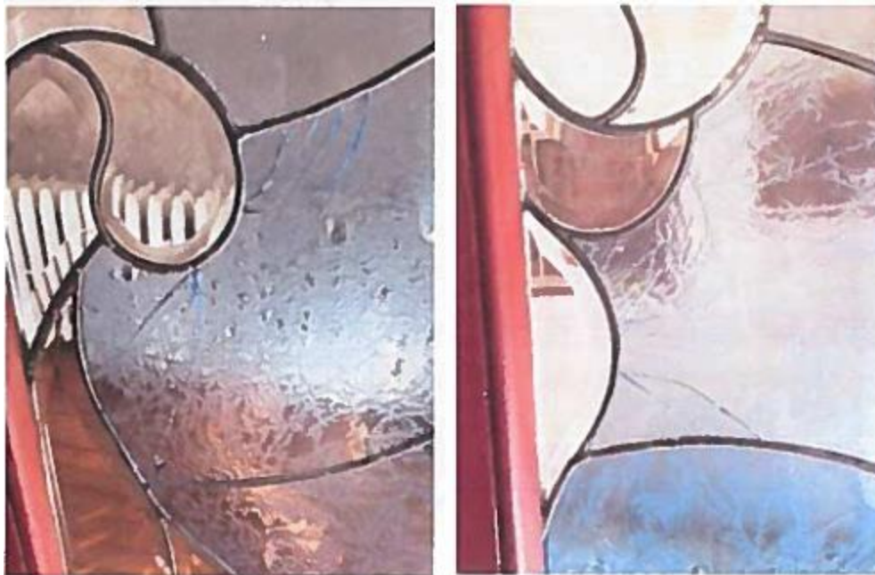
Stained glass removed, replaced with clear tempered glass.
