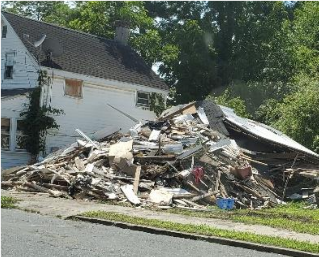
403 Pine Street – House Demolished
