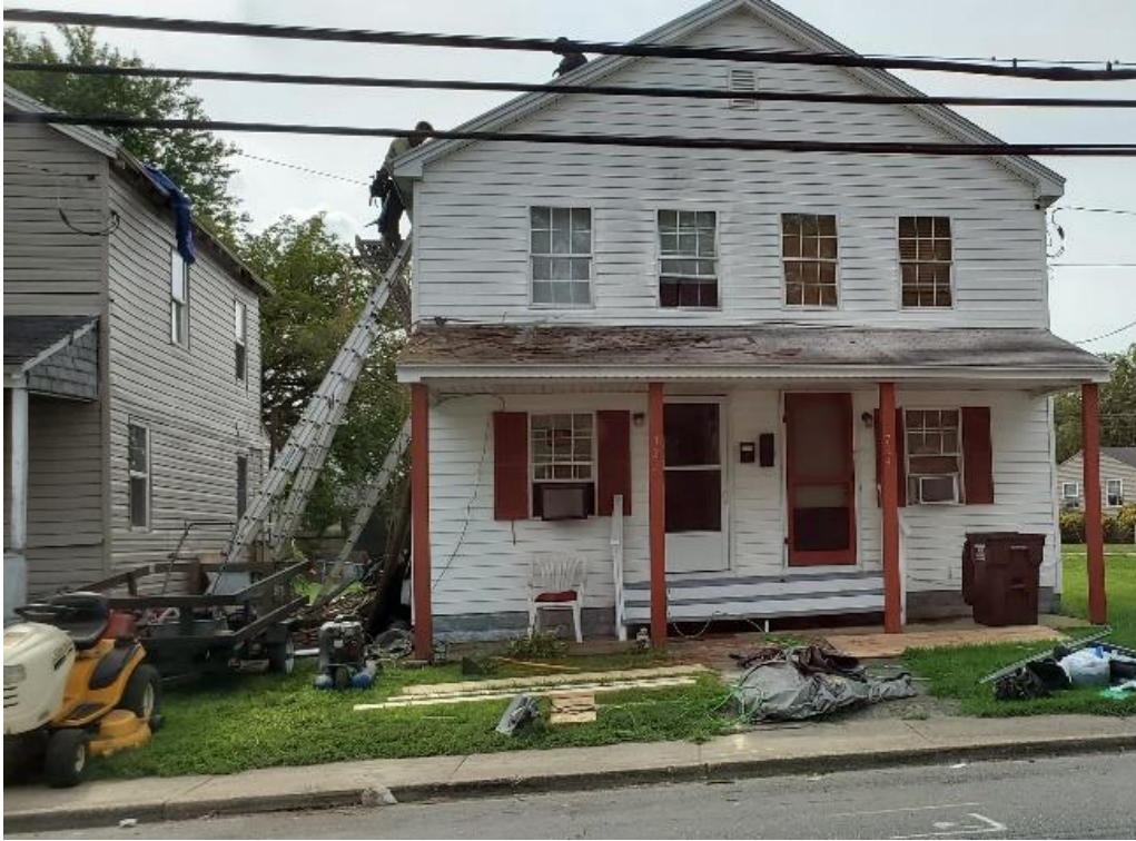
722 and 724 High Street – New Roof
