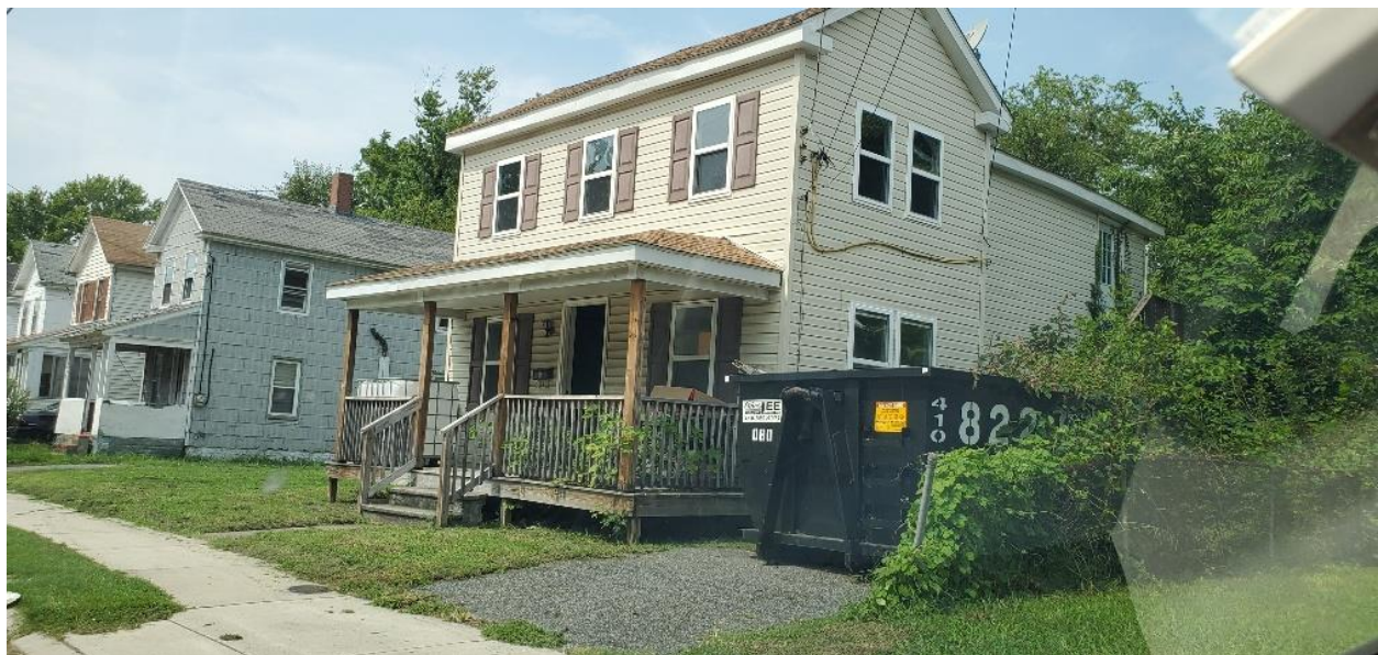
723 Washington Street – Interior Renovations
