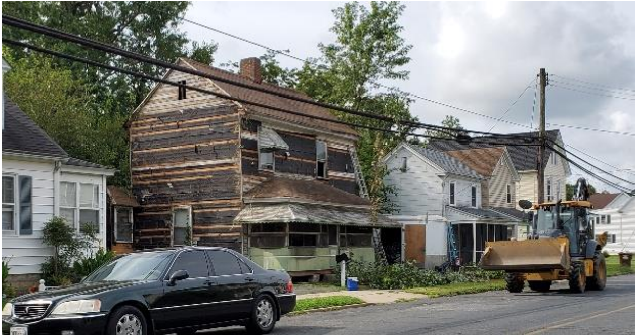
522 High Street – Abestos Shingles Removed – Ready for Demolition
